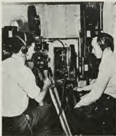
IN THE EARLY DAYS OF "TALKIES", CAMERAS WERE SO NOISY THAT THEY WERE ENCLOSED IN SOUND-PROOFED CABINETS, SHOWN BELOW AT RIGHT, IN A 1927 VITAPHONE STUDIO. THE CRAMPED QUARTERS OF A CAMERA BOOTH OF THAT ERA ARE PICTURED AT THE LEFT.
