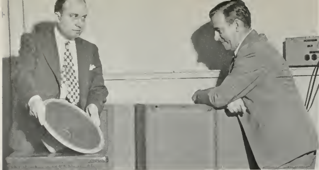
DR. H. F. OLSON (LEFT) AND J. PRESTON EXAMINE A DUO-CONE SPEAKER WHICH REPRODUCES THE COMPLETE AUDIBLE RANGE OF SOUND.
