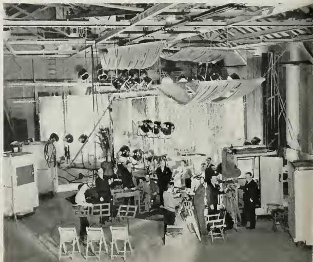
IN THE EARLY DAYS OF "TALKIES", CAMERAS WERE SO NOISY THAT THEY WERE ENCLOSED IN SOUND-PROOFED CABINETS, SHOWN BELOW AT RIGHT, IN A 1927 VITAPHONE STUDIO. THE CRAMPED QUARTERS OF A CAMERA BOOTH OF THAT ERA ARE PICTURED AT THE LEFT.
